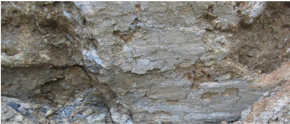
Photo 8. A view of fault outcrop at Çiftlikkale
