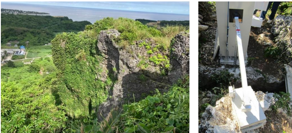
Photo 1: A view of a dangerous cliff in Miyagi Island of Okinawa Prefecture and its monitoring
