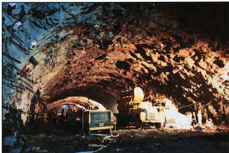
Top heading of cable bolted excavation in heavily bedded sandstone.
