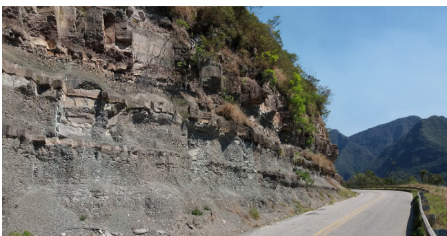
Fig. 1 Typical slope stability problem associated to slaking rock. (Source: Photo taken by the author).
