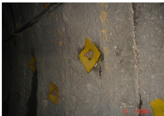
Fig 3. View of damaged and overstressed tunnel lining, with cracks in the shotcrete and deformed anchor plates. (Source: Photo taken by the author).
