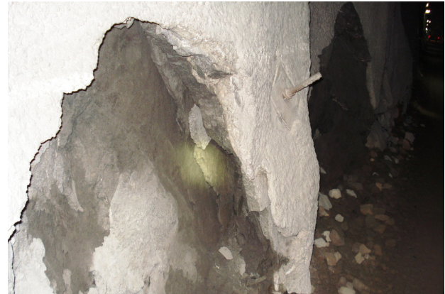
Fig 5. Partial failure of tunnel lining due to degradation. (Photo: personal file of the author).
