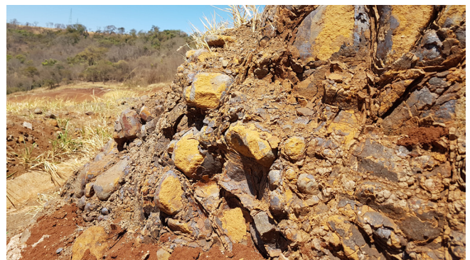
Fig. 2. Slaking basalt in a road cut generating stability and erosion problems. (Source: Photo taken by the author).
