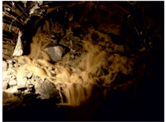
Fig. 10 : Heavy Flow of Water and Weak Rock
