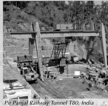
Pir Panjal Railway Tunnel T80, India
