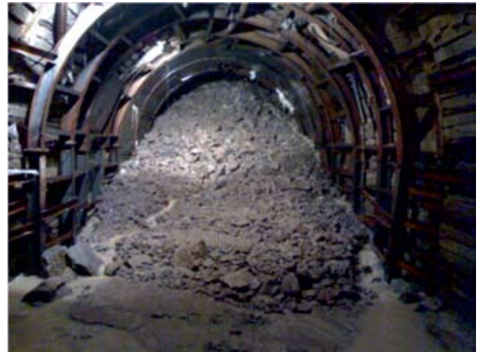
Fig. 3 : Extremely Weak Rock Creating Flowing Strata
