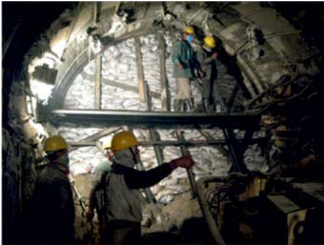
Fig. 6 : Plugged Face with Sand Bags
