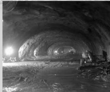
Strategic Crude Oil Storage Project in Underground Rock Caverns, India
