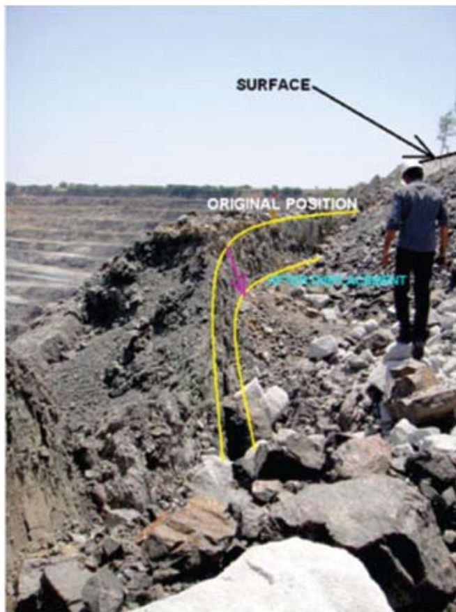
Photo 6 : Displacement of bench due to major fractures showing original position and after subsidence.
