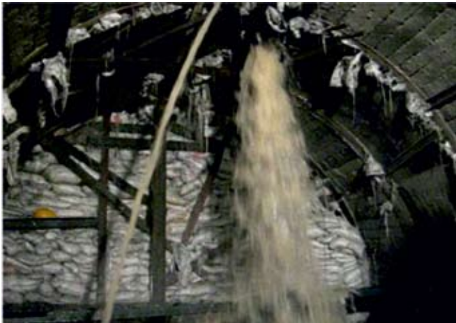
Fig. 4 : Plugging of Face with Sand Bags and Reinforced with Steel Angles
