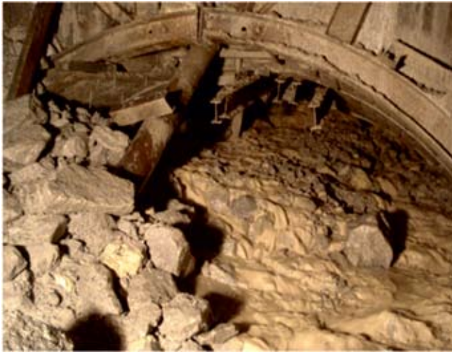
Fig. 2 : Flowing Weak Ground
