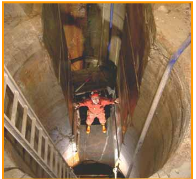
Figure 3. The boring of the two large holes formed the pillar. The pillar has been removed in five sawn blocks.
