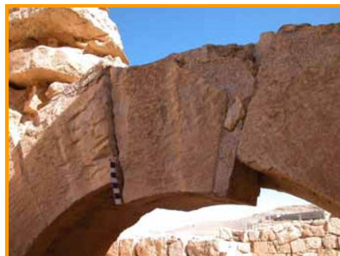
Figure 2. Preserved keyblock displacement in a Roman period arch at Mamshit (for location see Figure 1)
