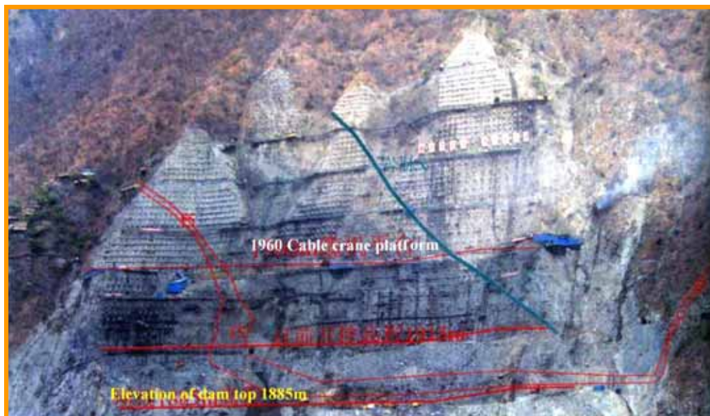
Figure 3. Overview of the slope on the left bank under construction
