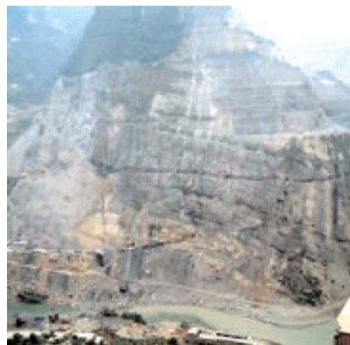
The Shuibuya Hydroelectric Project
